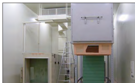
Air Volume Measurement Room
